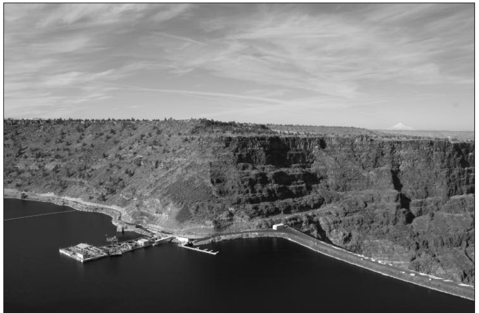
Completed in 1964, Round Butte Dam created Lake Billy Chinook. The collection and selective water withdrawal facility is at left. Photo by Jim Yuskavitch
