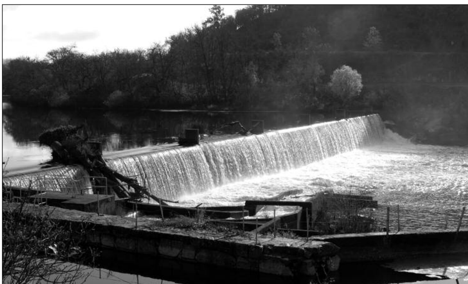
Ceasing to produce hydropower in 1972 due to obsolete generating facilities, the Gold Ray Dam was a liability to Jackson County, which owned it. The dam was removed in 2010. Photo by Jim Yuskavitch
